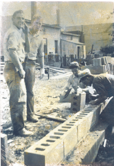
Norb, Eugene, and Ed Lodermeier, along with Bernard Gadiant laying the foundation for Lodermeier's Inc.
