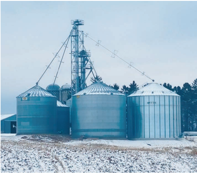
Dohrn Farms Kenny and Vicky Dohrn of Lake City, MN made a purchase of a new Brock bin for their farm to store more corn. The bin is 48' diameter and has a capacity of 61,689 bushels. Features include a Brock Tri-Corr floor with Parthenon floor support, a Sudenga 8" Clean Sweep, 10hp low-speed centrifugal fan, and roof vents.
