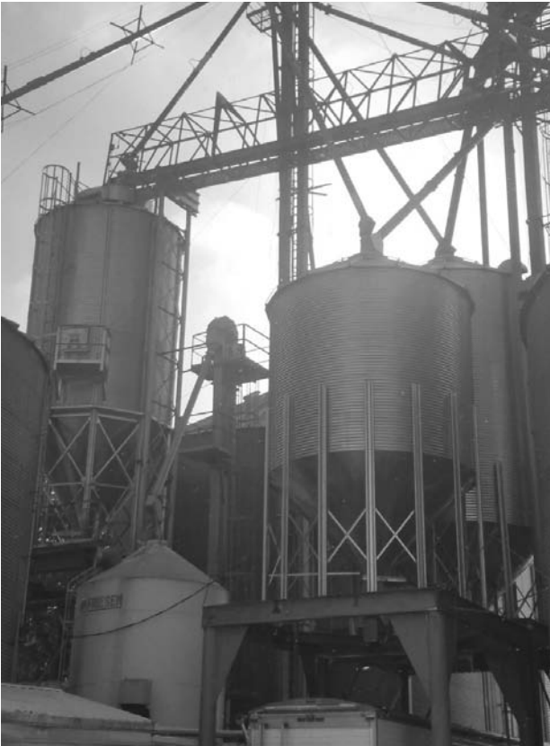
Rostad Farms Joel and George Rostad of Zumbrota, MN called Lodermeier’s with a need to replace several overhead hopper bins on their grain site. Our crew put our crane service to work and took down all three bins and replaced them with new Brock 15’ hopper bins. Two of the bins were ordered with 60 degree cones for better unloading.
