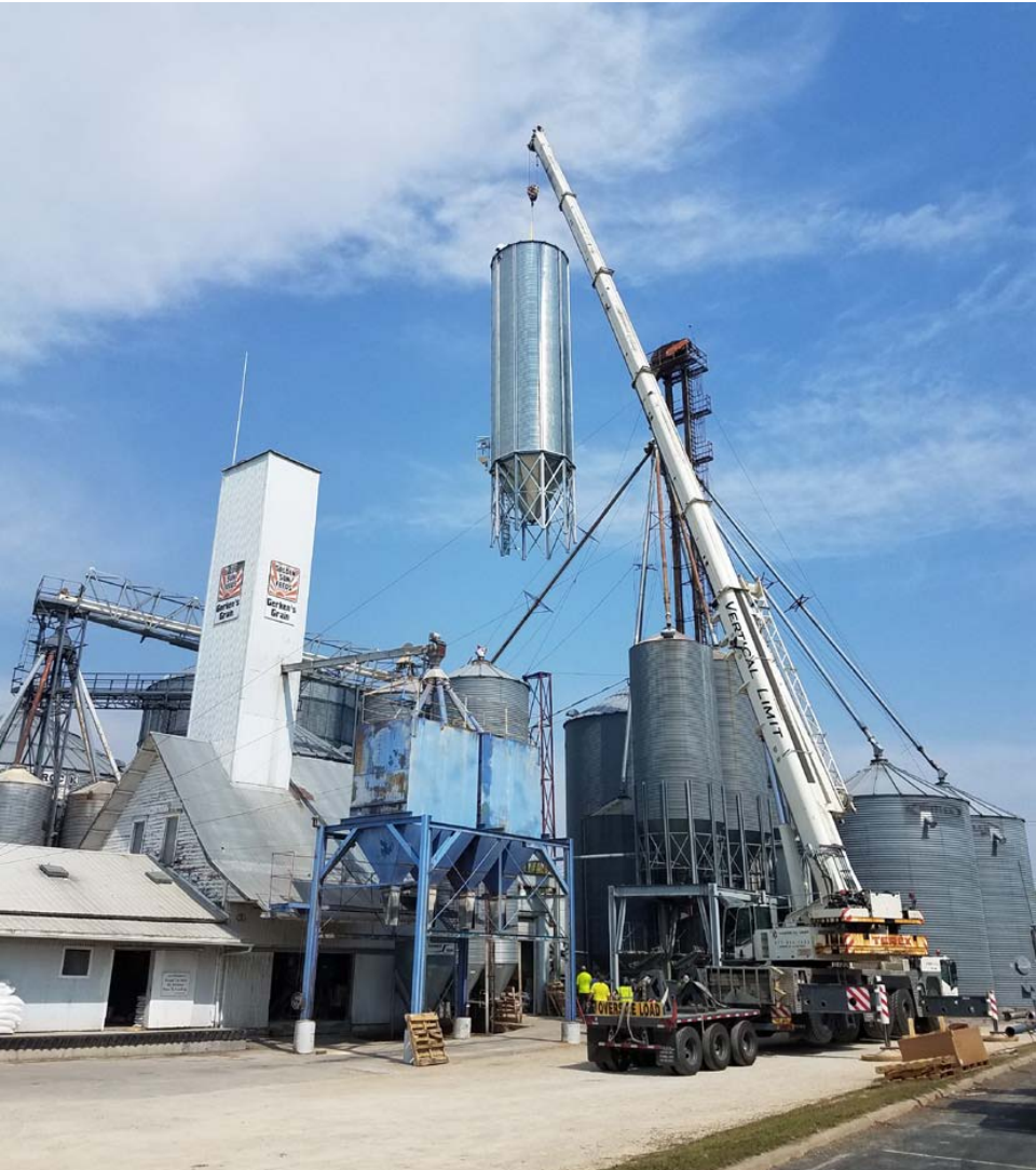
Gerken Feed and Grain Zumbrota's Gerken Feed and Grain contacted Lodermeier's with the need to replace a wet holding bin. The decision was made to go with a taller bin and get rid of the old one. A new Brock 15' diameter x 17-ring commercial E-Series bin was constructed and installed with the help of Vertical Limits Crane Service. The bin has a 60 degree hopper bottom, commercial roof, and sidewall access door.
