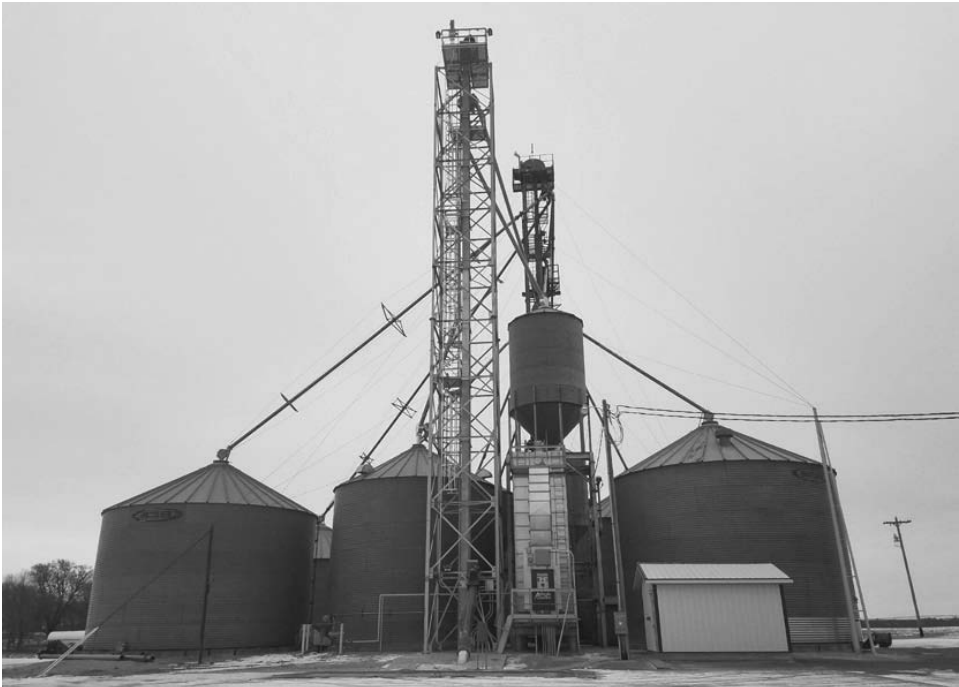
Randy Kimmes Randy Kimmes of Hastings, MN worked with Lodermeier’s to design a new grain unloading area at his grain site. Lodermeier’s crew installed a new Hyland Grain Systems 975 bushel pit. The pit features a 10’ x25’ dump-through grate and a 14” x 5,000 bph auger. Then a new Hyland Grain Systems leg and tower were installed. The leg and tower stand 100’ tall and are built of galvanized material. The leg feeds the wet bins and dryer.
