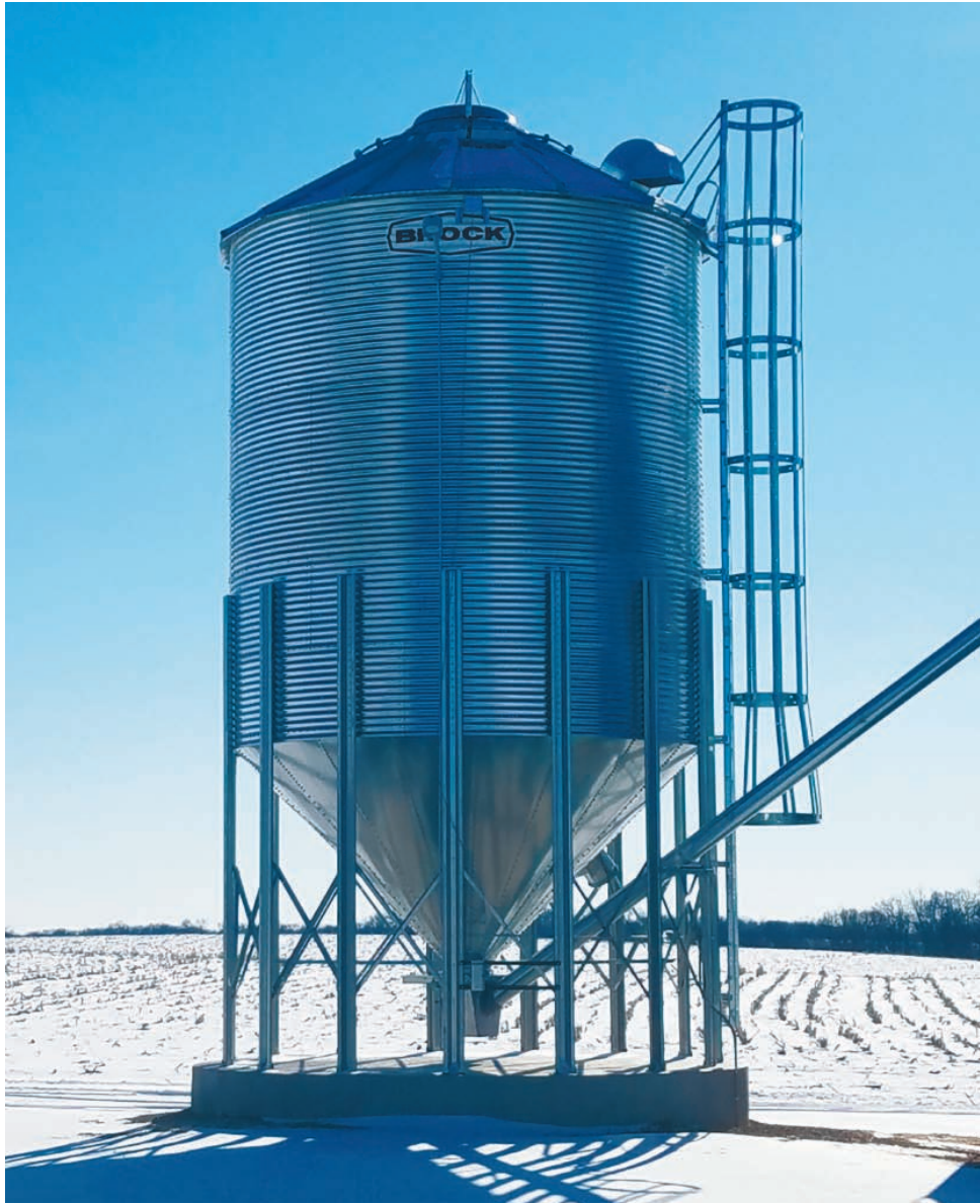
Howard Larson Howard Larson of Pepin, WI contracted with Lodermeier's to increase his wet holding capacity. He went with a new Brock 15' diameter x six-ring hopper bin with a capacity of 2,925 bushels. The bin included a 12" axial fan for aeration, an Access Plus hopper door and a ground operated lid.
