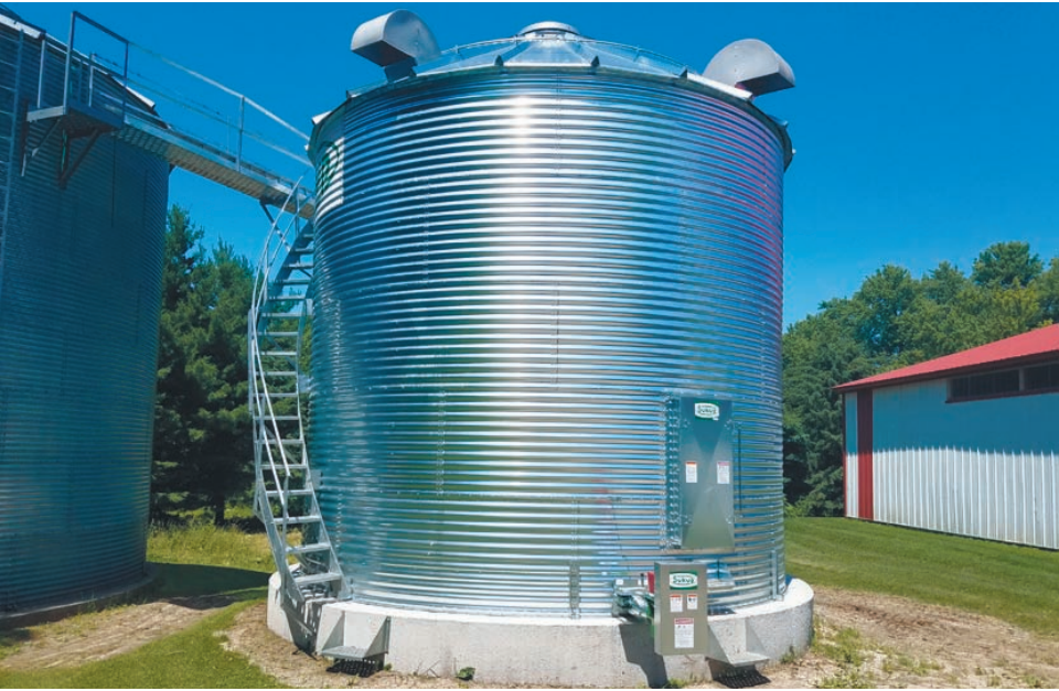
Mike Ruprecht Mike Ruprecht of Lewiston, MN chose to have Lodermeier's construct a new Sukup 21' diameter x 18' eave bin with a capacity of 5,614 bushels. The bin has four poly vents, small grain floor, axial fan, Greene Stairway, and 8" Sukup powersweep.
