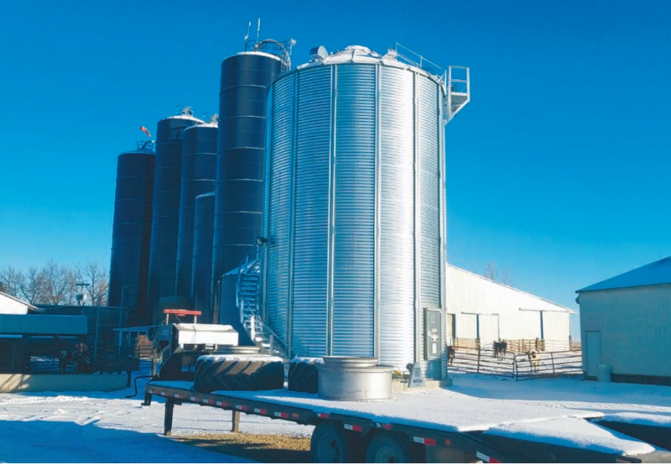
Kurt Ronningen Kurt Ronningen of West Concord, MN worked with Lodermeier’s to add a new Brock storage bin to his farm site. The bin holds 9,841 bushels and includes a Shur-Step outside stairway, roof handrail, 8” powersweep unload and a 5hp high-speed centrifugal fan. Kurt built this bin himself along with some help.
