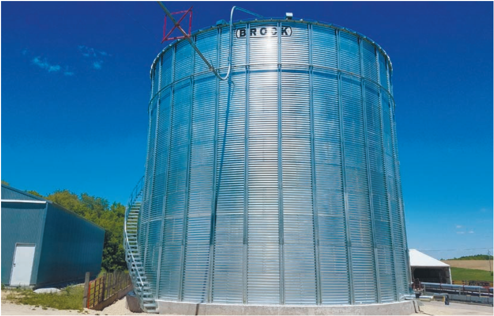
Tom and Tanner Ferrier Tom and Tanner Ferrier of Dover, MN contacted Lodermeier’s with the request for more grain storage. After talking it over they decided to construct a Brock 48’ diameter x 40’ eave bin with an approximate capacity of 66,275 bushels. The bin has a Brock Tri-Corr floor with Parthenon floor supports, and 15hp low-speed centrifugal fan, Sudenga 8” Clean Sweep, and a Shur-Step stairway.
