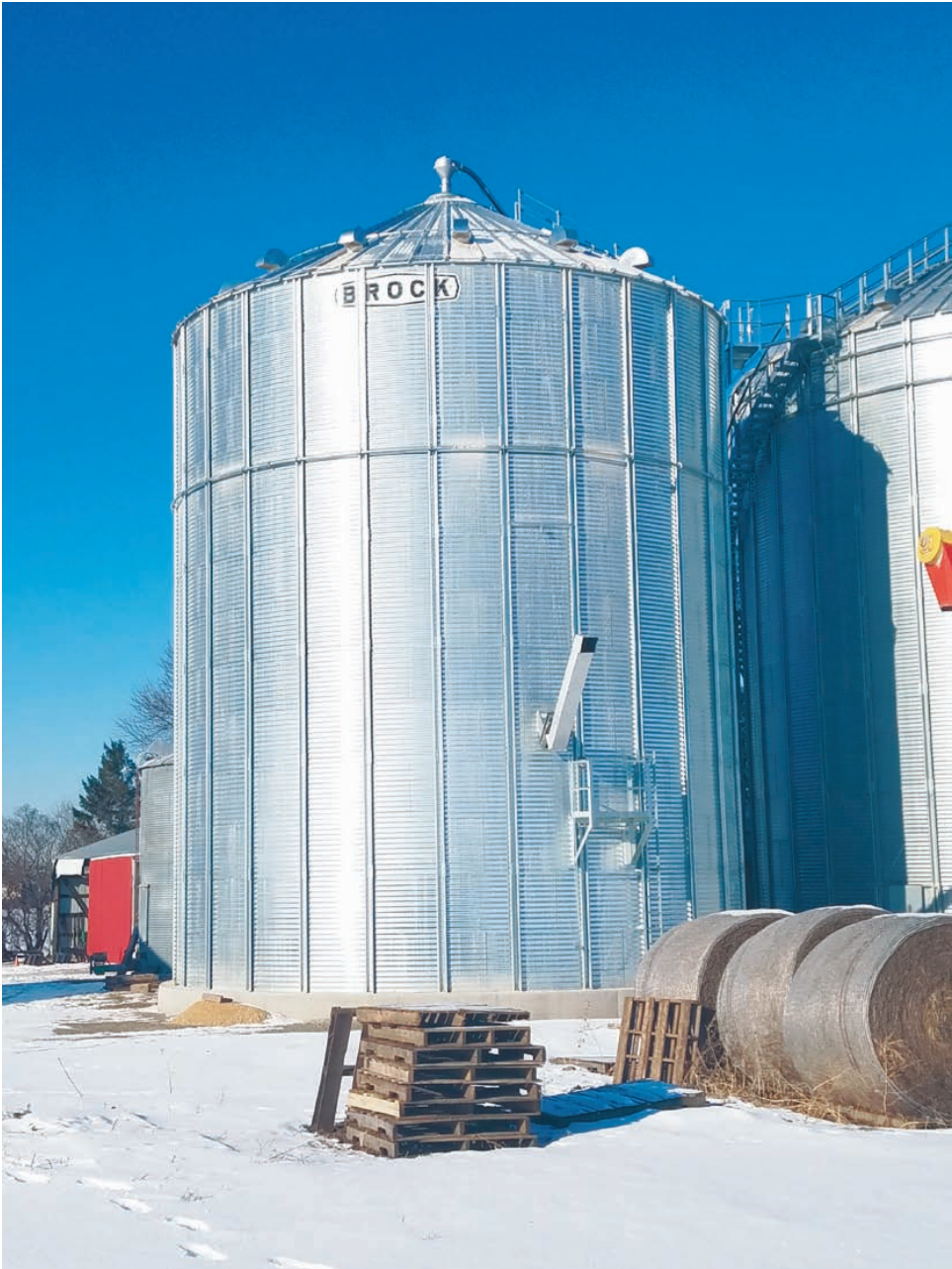
Ron Schiltgen Ron Schiltgen of Afton, MN contracted with Lodermeier’s to replace two bins at his farm in 2017. First we installed a new Brock 18’ diameter x eight-ring wet holding hopper bin with a capacity of 5,514 bushels. The bin included a roof handrail, Access Plus hopper door and Levalert bin full indicators. The second bin Schiltgen went with was a Brock 42’ diameter x 48’ eave bin with a capacity of 58,700 bushels of dry corn. Some of the features included a 10” powersweep unload, fifth-ring side load out and a custom built catwalk to connect to his existing 48’ Brock bin as well.
