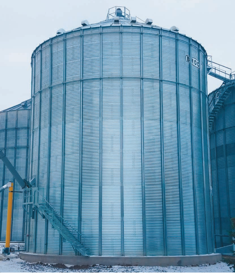
Erickson Farms Jeff and Todd Erickson found themselves going into fall short of corn storage. They made the decision to purchase a new Brock 48' diameter x 51' eave bin. This bin has a capacity of 83,036 bushels. This bin is loaded up with great features including low-speed centrifugal fans, Sudenga 10" Clean Sweep with a 12" vertical powerhead, a shared Shur-Step stairway with another side-by-side bin, side draw with hinged spout, Brock Tri-Corr floor aeration, and Boone temperature cables.
