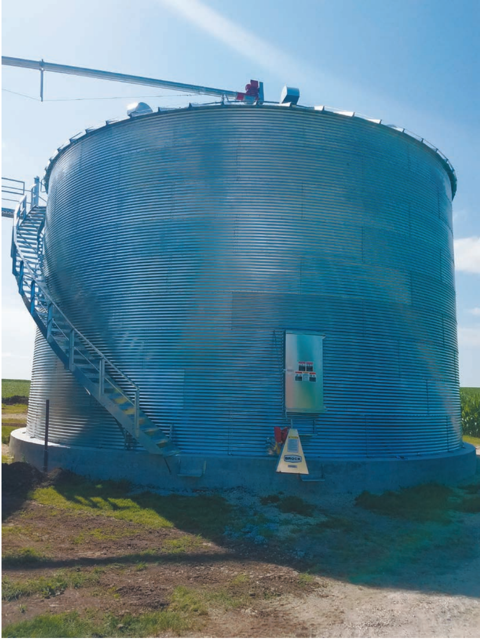
Terry Engler Terry Engler of Elgin, MN contracted with Lodermeier’s to construct a new Brock 42’ diameter x nine-ring bin with a capacity of 31,056 bushels. The bin has a Tri-Corr floor with Parthenon floor supports, Sudenga 8” Clean Sweep, Shur-Step stairway, low-speed centrifugal fan, and electric grain spreader.
