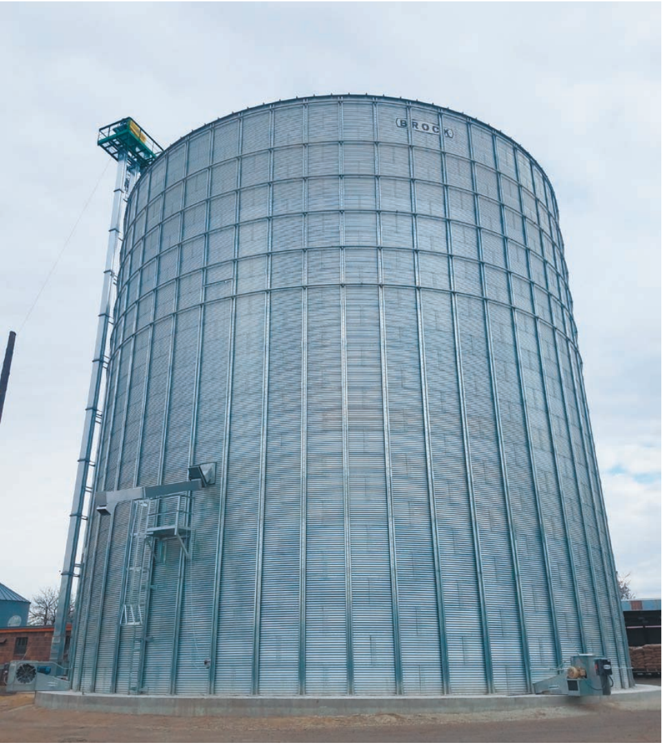
Gerken Feed and Grain Wabasha's Gerken Feed and Grain purchased a new grain bin from Lodermeier's to hold this year's bumper crop. A new Brock 78' diameter x 28-ring Commercial E-Series bin with 323,852 bushels of storage was erected at the elevator. The bin includes a Brock Tri-Corr floor with Parthenon floor supports, a Hutchinson 10" powersweep, sidedraw unloading with a hinged spout, three Brock high-speed centrifugal fans, and Brocks commercial roof.
