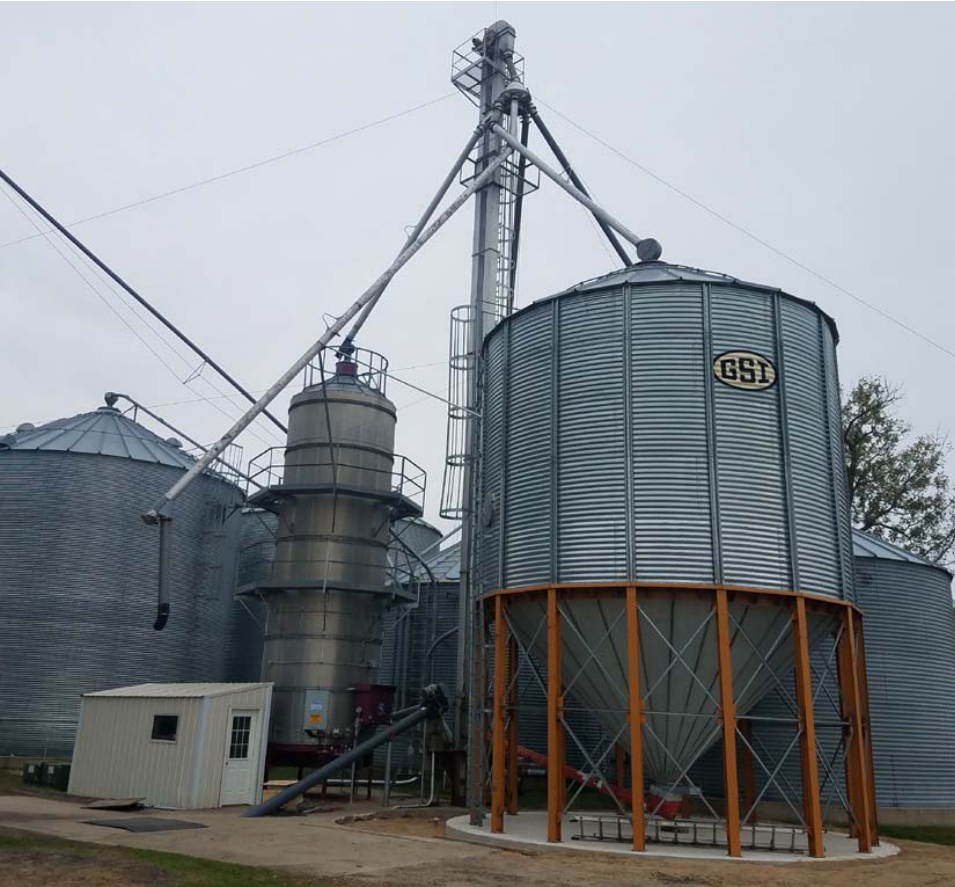
Dan Erickson Dan Erickson of Alden contacted Lodermeier’s interested in a used MC dryer. After some discussion they hired a Lodermeier’s crew to install the used MC 10730 continuous flow dryer. Lodermeier’s also installed a new Jemco 40hp VariAir grain transfer system. The grain transfer system has a VFD control for easy operation.
