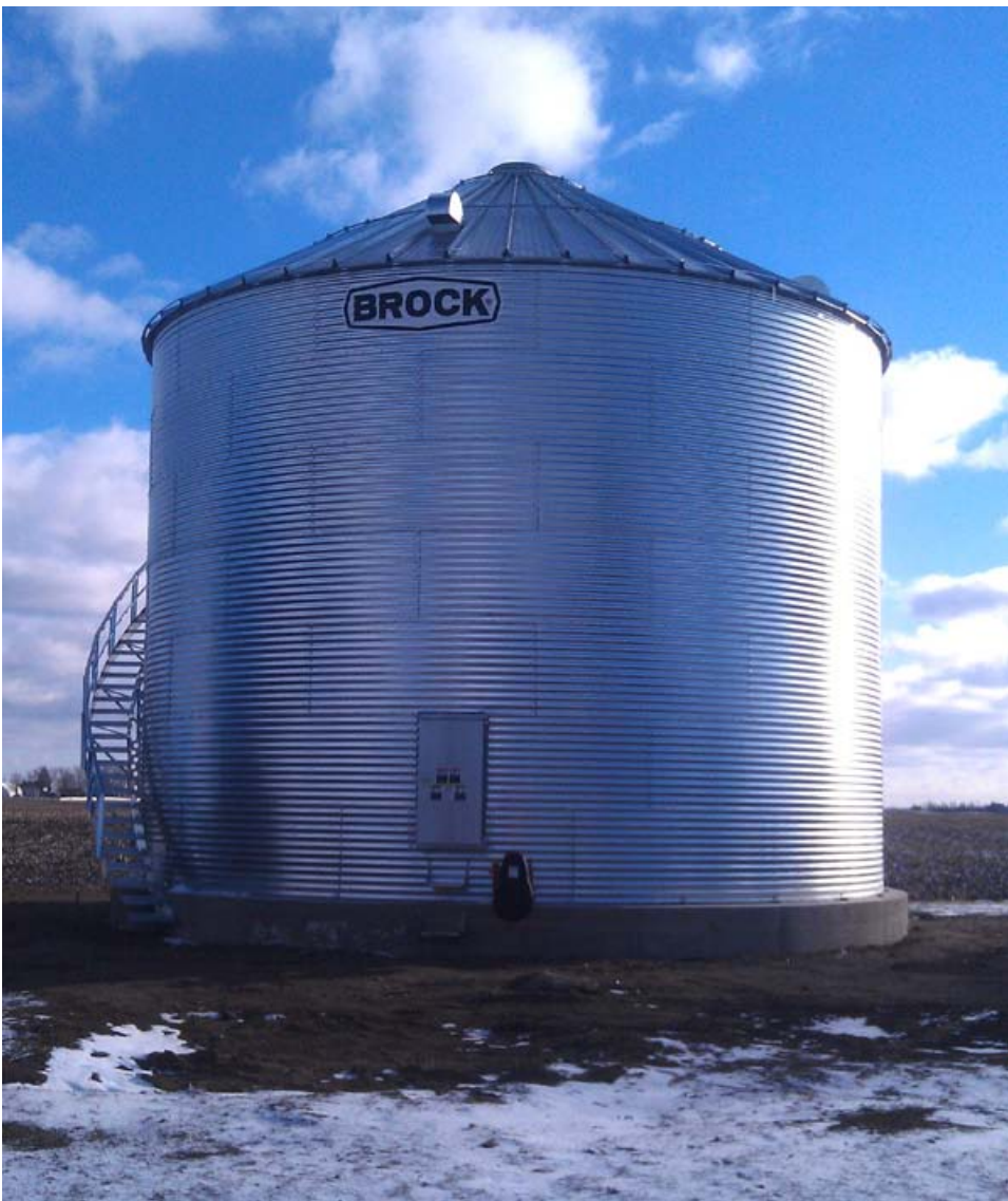
Ruth Kiihbauch Ruth Kiihbauch of Hastings, MN hired Lodermeier's to construct a new Brock 36'x26' bin. The bin has a capacity of 23,765 bushels. A Tri-Corr floor with Parthenon floor supports, an 8" powersweep and a Shur-Step stairway were installed on this bin.
