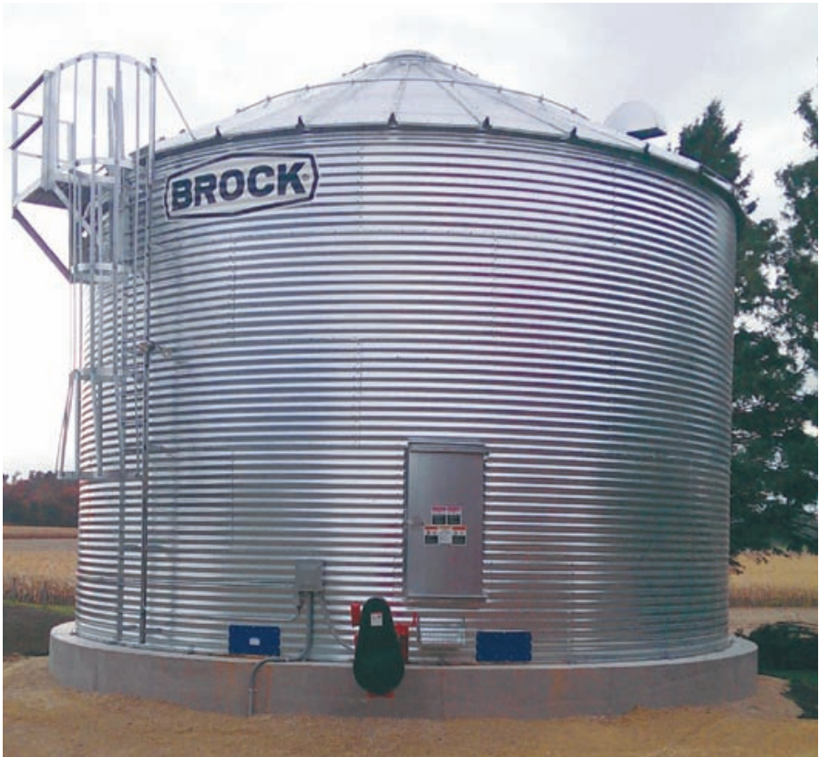
Curt Meyer Curt Meyer of Lake City, MN hired Lodermeier’s to build a new Brock 30’ x 18’ storage bin. The bin has a 10” powersweep unload, Tri-Corr floor with Parthenon supports, 24” 5hp axial fan and six roof vents.
