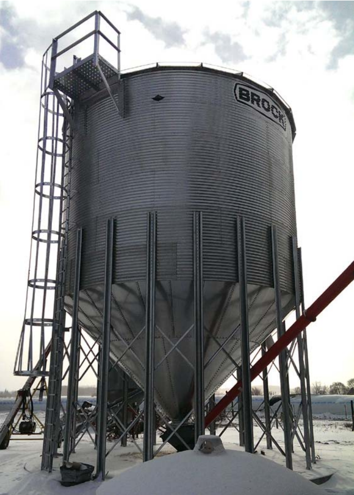
Tom Leisen Tom Leisen of Plainview, MN hired Lodermeier's to construct a new wet holding bin on his farm. Tom went with a Brock 21' diameter x 6 ring tall bin with a capacity of 6,100 bushels. The bin included an outside ladder, two roof vents and an Access Plus hopper door.
