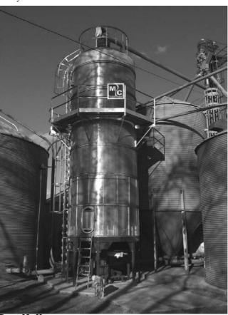
Liebenow purchased a Brock 48' diameter x 40' eave with continuous flow tower dryer. The dryer has aluminum outer storage capacity of 66,000 bushels. The bin included a Brock screens, new moisture sensing, sloped inner floor, and a
