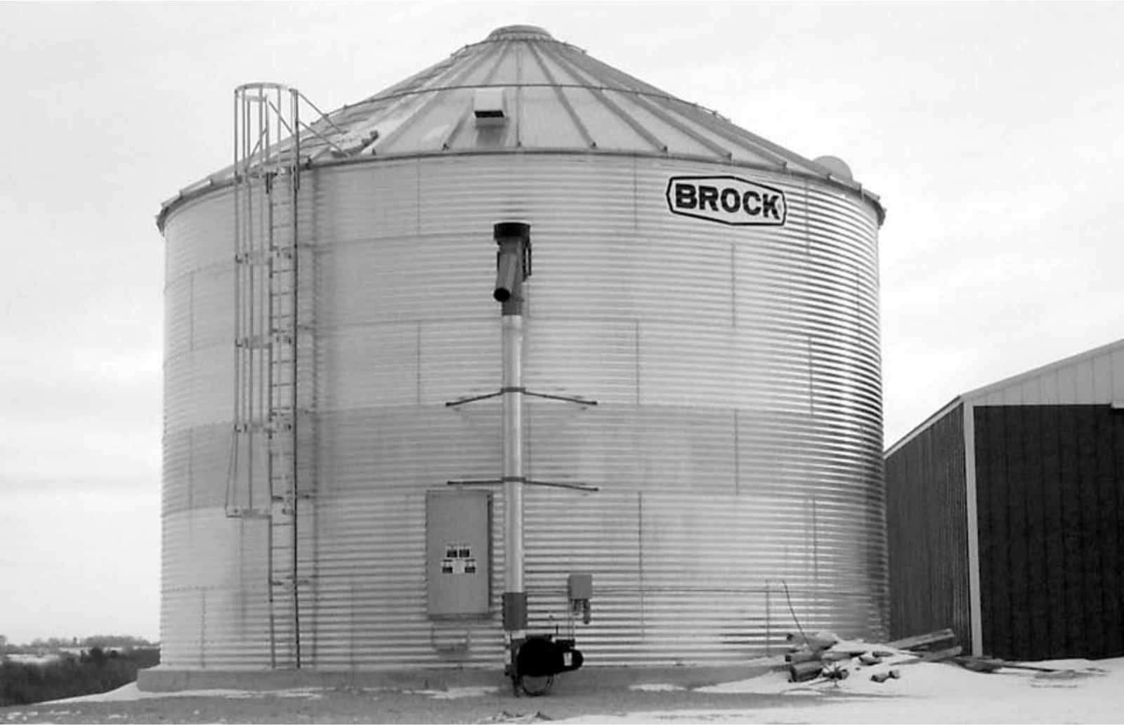
DENNIS HINSCH Dennis Hinsch of rural Goodhue, MN contracted with Lodermeier's to put up this 36' x 22' Brock grain storage bin. /this bin features 4 roof vents, Brocks Tri-Corr floor and Parthenon supports, 8" powersweep with a 16' x 10" vertical auger and an 18" axial fan and transition.
