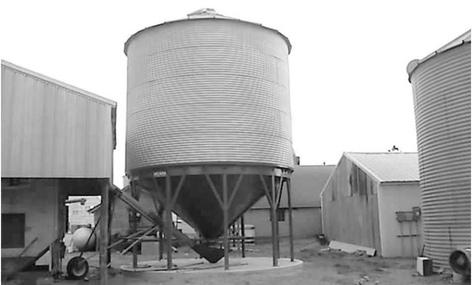
NICK PEINE Nick Peine from Hampton, MN purchased this 18' Micada hopper for his 18' storage bin, thereby converting it to a hopper bin for wet corn. Nick did all the work himself.
