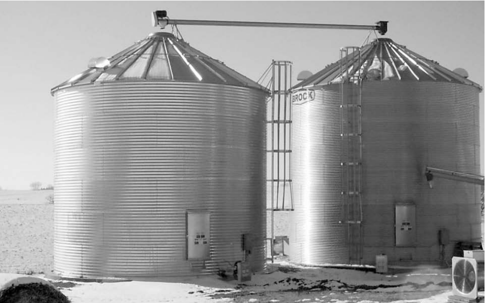
KEVIN, HENRY AND CRAIG THOMFORDE Kevin, Henry and Craig Thomforde purchased this 27' x 22'. Brock grain storage bin from Lodermeier's. The Thomfordes built the bin themselves and had Lodermeier's install the 8" powersweep, and then the Thomfordes installed the Tri-Corr floor and Parthenon supports. This bin also has an 18" axial fan and 2 roof vents.
