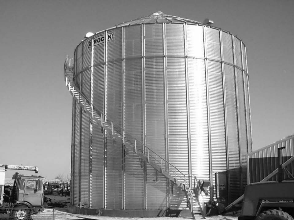
BRUCE ALBERS Bruce Albers of Goodhue, MN purchased a Brock 48'x40' grain bin. This bin features sidewall stairway, full floor aeration, 8" power sweep and 2nd tier side draw.
